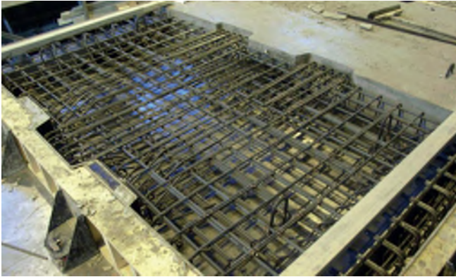
Figure A.5 Production of a match-cast concrete deck element for a large-scale test specimen
