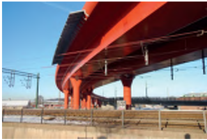
(a) Composite bridge over railway
