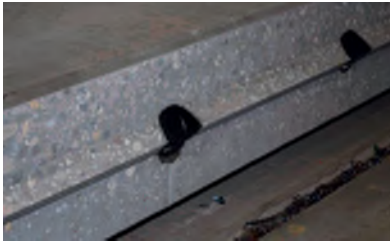
(b) Dry joints with linear shear keys, Germany (Möller et al. 2012a)
