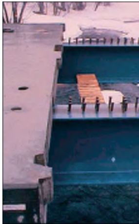
(c) Bridge deck element in final position
