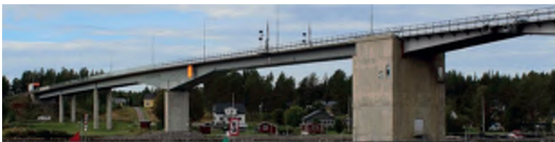
(c) The Pitsund Bridge in Piteå (Sweden)
