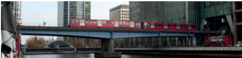
(a) Docklands Light Railway bridge in London (UK)
