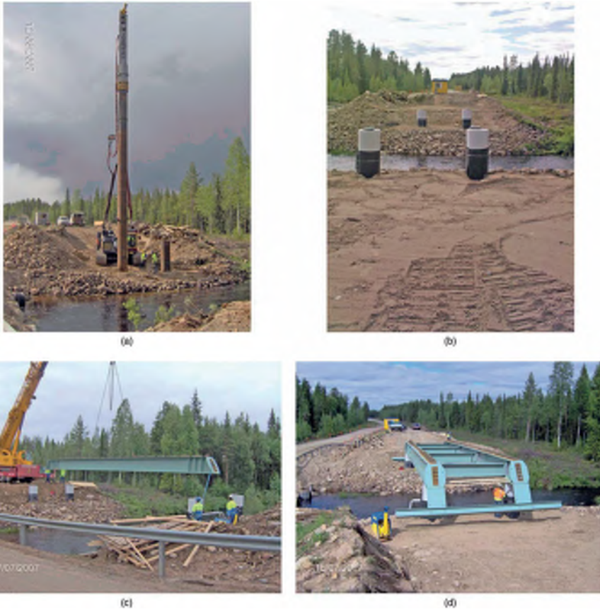
Fig. 13. Construction sequence for the Laisentiajoki bridge (Reprinted with permission from Harju 2009): (a) large diameter steel piles being driven into the soil; (b) concrete filled piles with bearings in place; (c) steel girders being lifted into place; (d) completed steel structure; (e) prefabricated concrete end beams and wing walls being placed into final position and cast to the steel girders; (f) erection of prefabricated concrete deck elements; (g) prefabricated deck placed and awaiting concrete closure pour; (h) composite action is achieved by in situ cast concrete in the open channels
