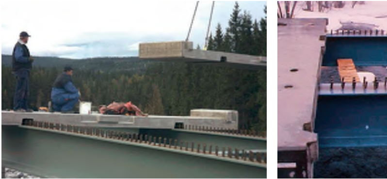
Figure 3.6 Erection of elements at the Norrfors Bridge (left) and the Rokån bridge (right)
