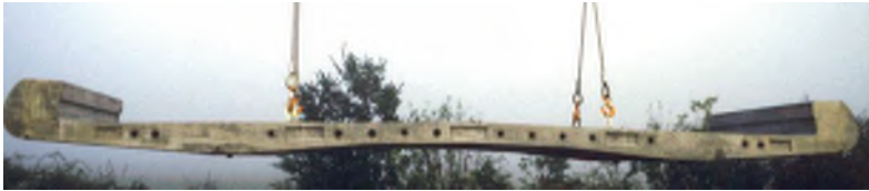
(a) Prefabricated bridge deck element with dry joints, France (Berthelley 2009)
