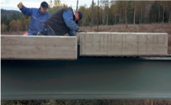
Figure A.7 Erection of a prefabricated concrete deck element
