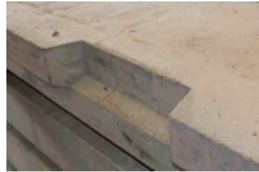
(c) Dry joints with overlapping concrete shear keys, Sweden (Hällmark 2012a)
