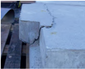
(a) Photo of the expected type of failure
