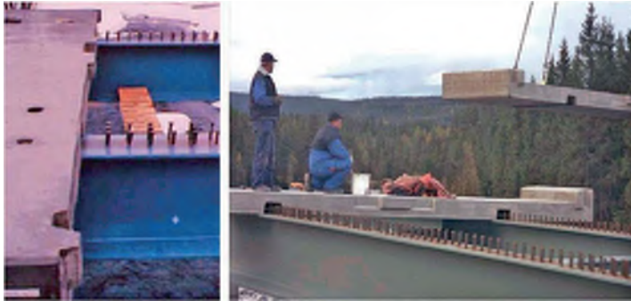
Fig. 14. Deck elements with dry joints (Reprinted with permission from Hällmark et al. 2009; first published in Structural Engineering International SEI , Vol. 19, Nr. 1, 2009, pp. 69–78, IABSE, Zurich, Switzerland, www.iabse.org )
