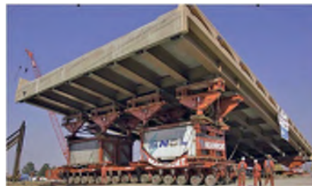
Fig. 4. SPMT transportation of 4500 South Bridge, Utah (Reprinted with permission from Mammoet USA South, Inc.)
