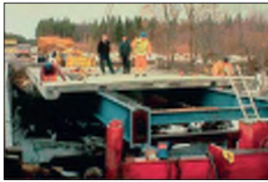
(a) Two more deck elements to go
