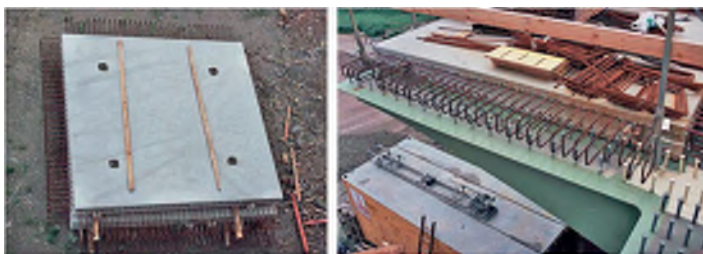
Fig. 9. Bahretal viaduct with prefabricated full-depth slab elements (Reprinted with permission from Seidl 2009)
