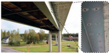
Fig. 4. Pitsund Bridge after postinstallation of CSPs.
