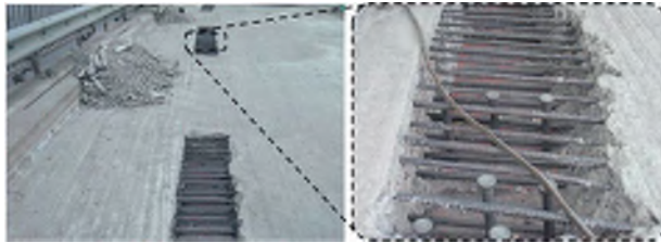
Fig. 2. Postinstallation of welded shear studs.
