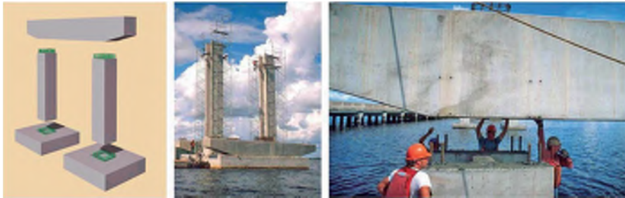
Fig. 6. Prefabricated substructures (FHWA 2009)
