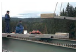
Fig. 18: Bridge deck element is lifted in place
