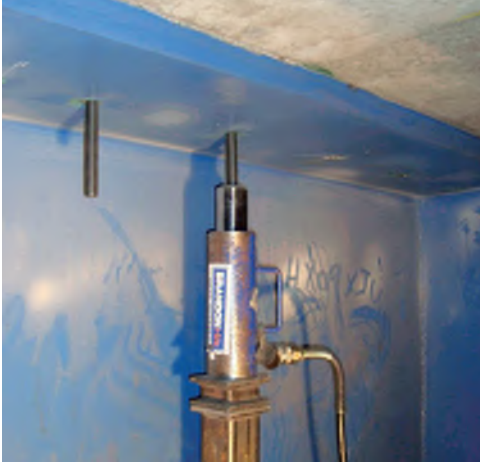
Figure 4.25 Installation of CSPs in the DLR-bridge
