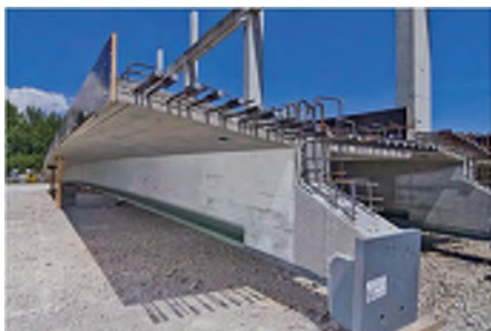
Fig. 8. Prefabricated VFT-girder (Reprinted with permission from Seidl and Braun 2009)
