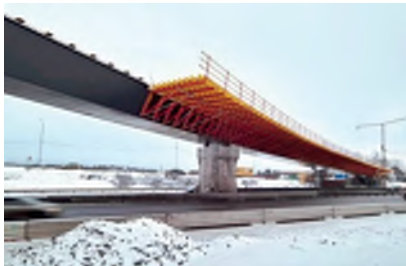
(c) Composite bridge over motorway
